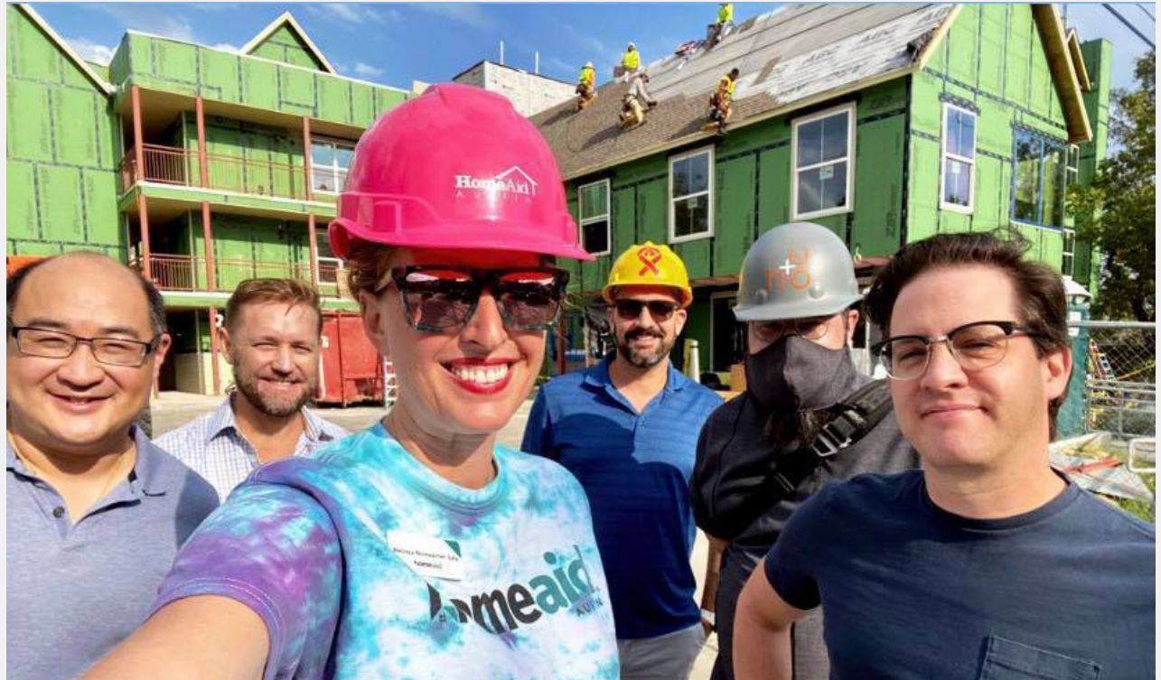
A group from HomeAid Austin constructs the new Hayes Caldwell Women's Transitional Housing project, which will feature donated Delta® fixtures.
